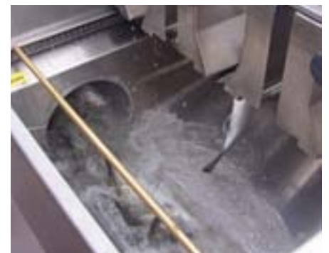
View into outlet hopper out of channels.
