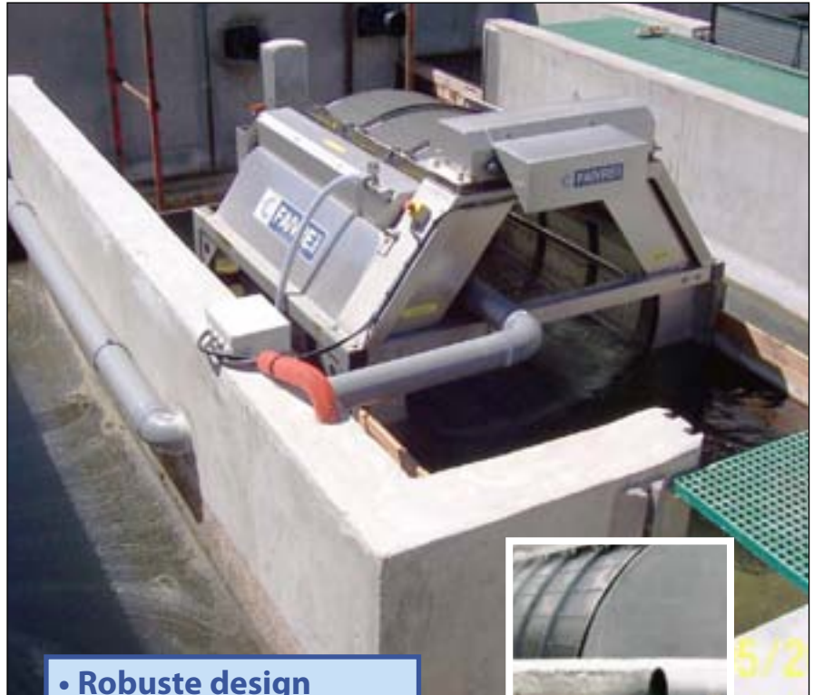
Filter 12-160 with frame on a fish farm outlet.
